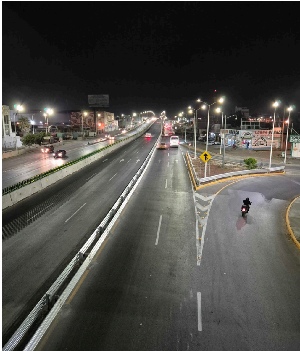
Paso Sup. Vehicular Central de Abastos
